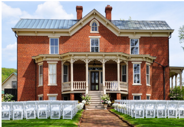
East facing side yard
